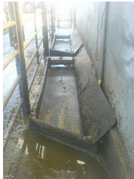
Fig 5: A well designed footbath with pre-wash and agent bath
