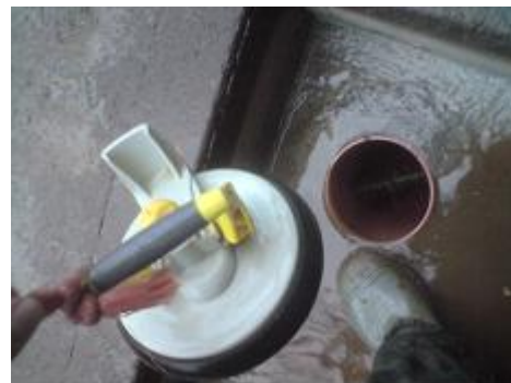
Fig 6: A 6" drain, bung and string pull.
